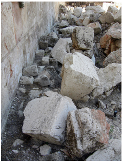
Rocks left after Temple Destroyed in 70 AD
